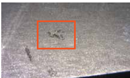
IMAGE 2: Example of fracturing and pit formation due to excessive startup friction
